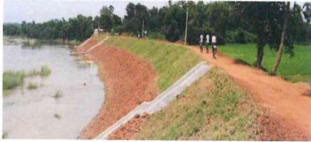
Figure 4- River plain with embankments
