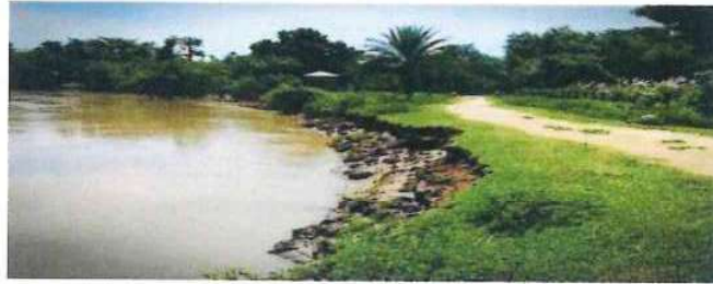
Figure 5 - River plain without embankments
